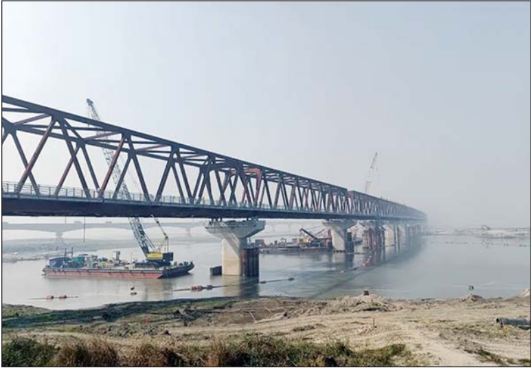
Under Construction rail bridge over the Jamuna river
