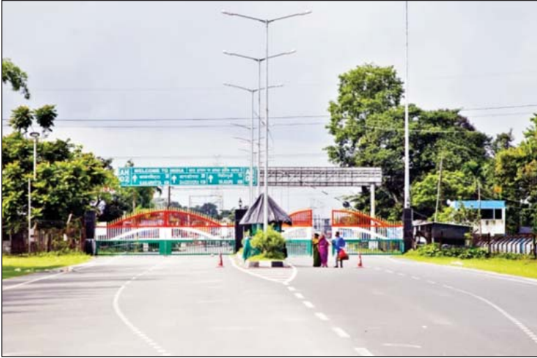
Newly constructed Banglabandha Land Part at Tetulia in Panchagarh
