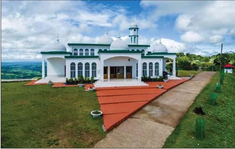
The Central Mosque at Sajek Valley, Rangamati
