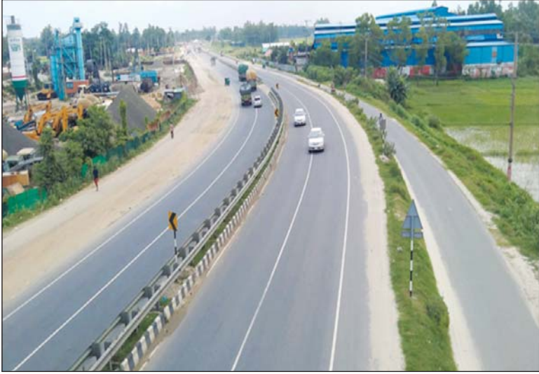
Newly Constructed Dhaka-Tangail Highway
